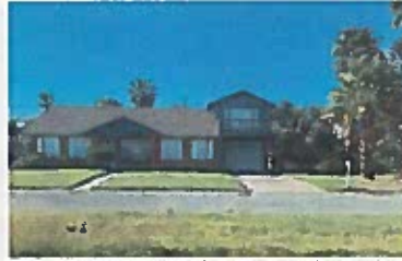
Figure 3.3: Single-family residence Picture Courtesy: Emily Tedford
