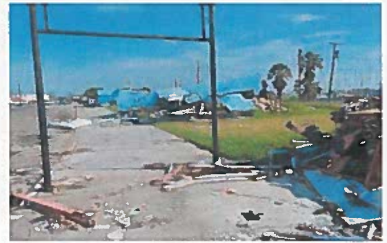
Figure 8.16: Hurricane Harvey's destruction of the Heritage District
