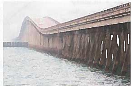
Figure 5.2: Copano Bay Bridge Source: static.tti.tamu.edu
