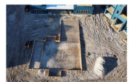
Swimming pool is framed and prepped for installation
