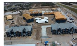
Phase 2 construction is 34% complete
