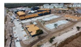
All building pads are in place and paving is 50% complete
