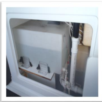
Potable Water Tank
