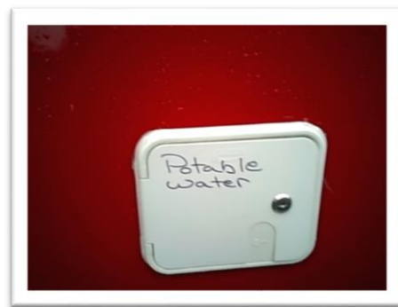
Potable Water Inlet
