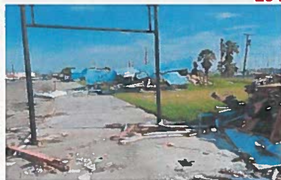
Figure 8.16: Hurricane Harvey's destruction of the Heritage District
