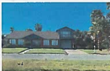
Figure 3.3: Single-family residence Picture Courtesy: Emily Tedford
