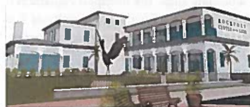
Figure 8.19: RCA Renovation Source: Dykema Architects, INC
