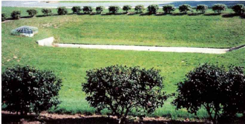
A detention basin in an urban area.
