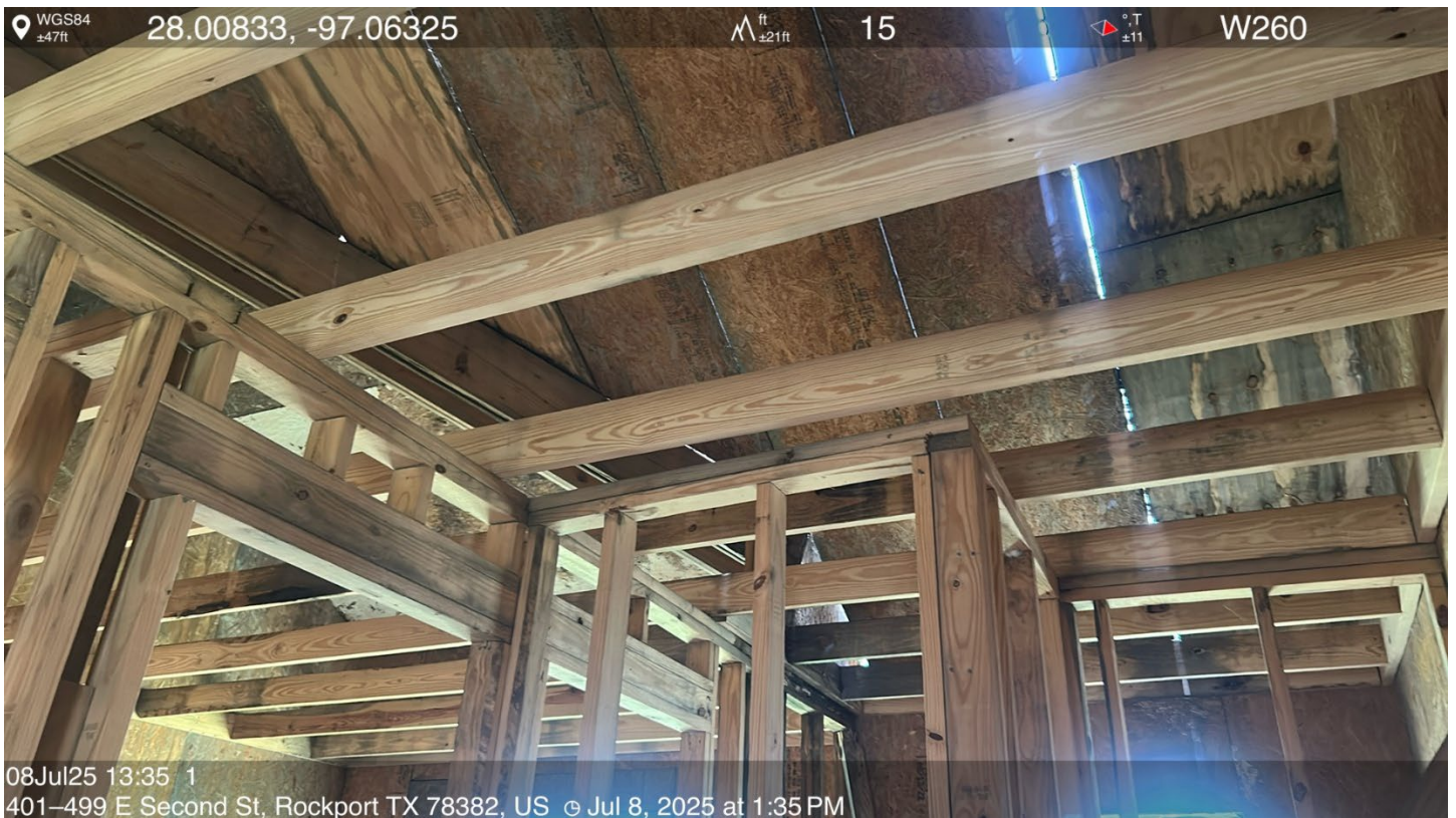
Water damage to 2 nd floor
