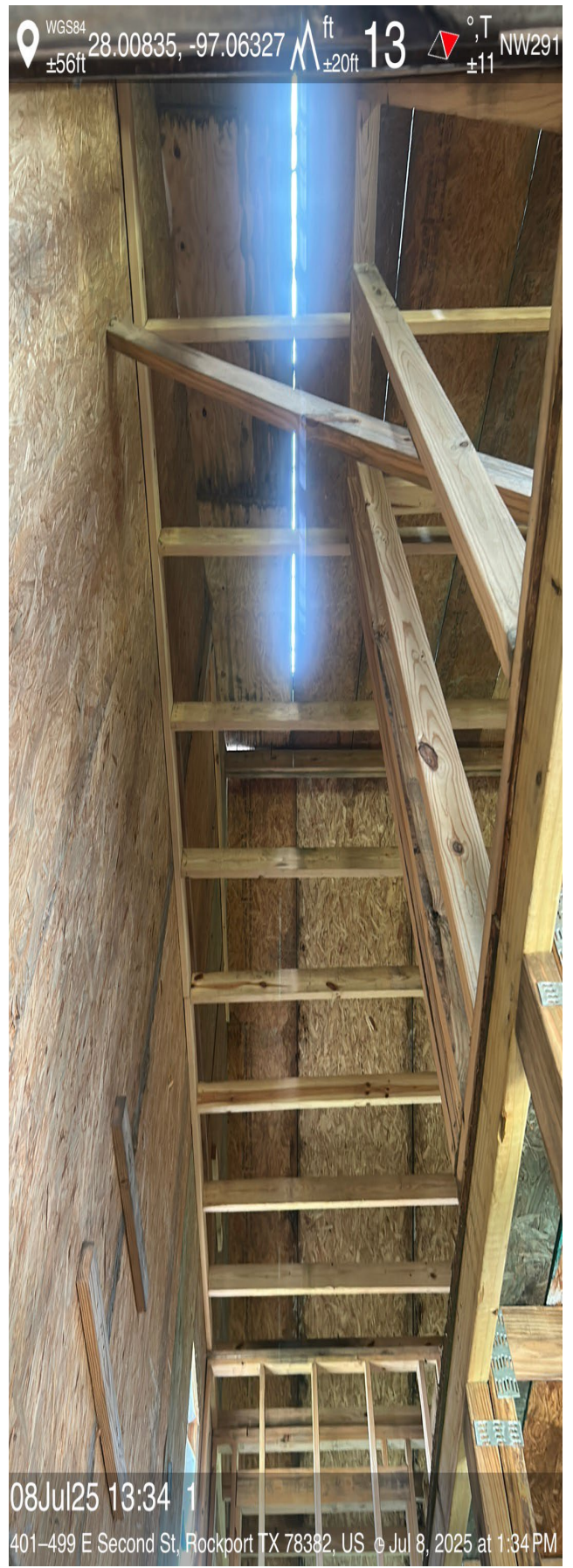
Spaces in Roof
