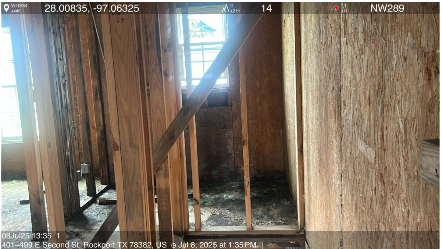
Water damage to 2 nd floor
