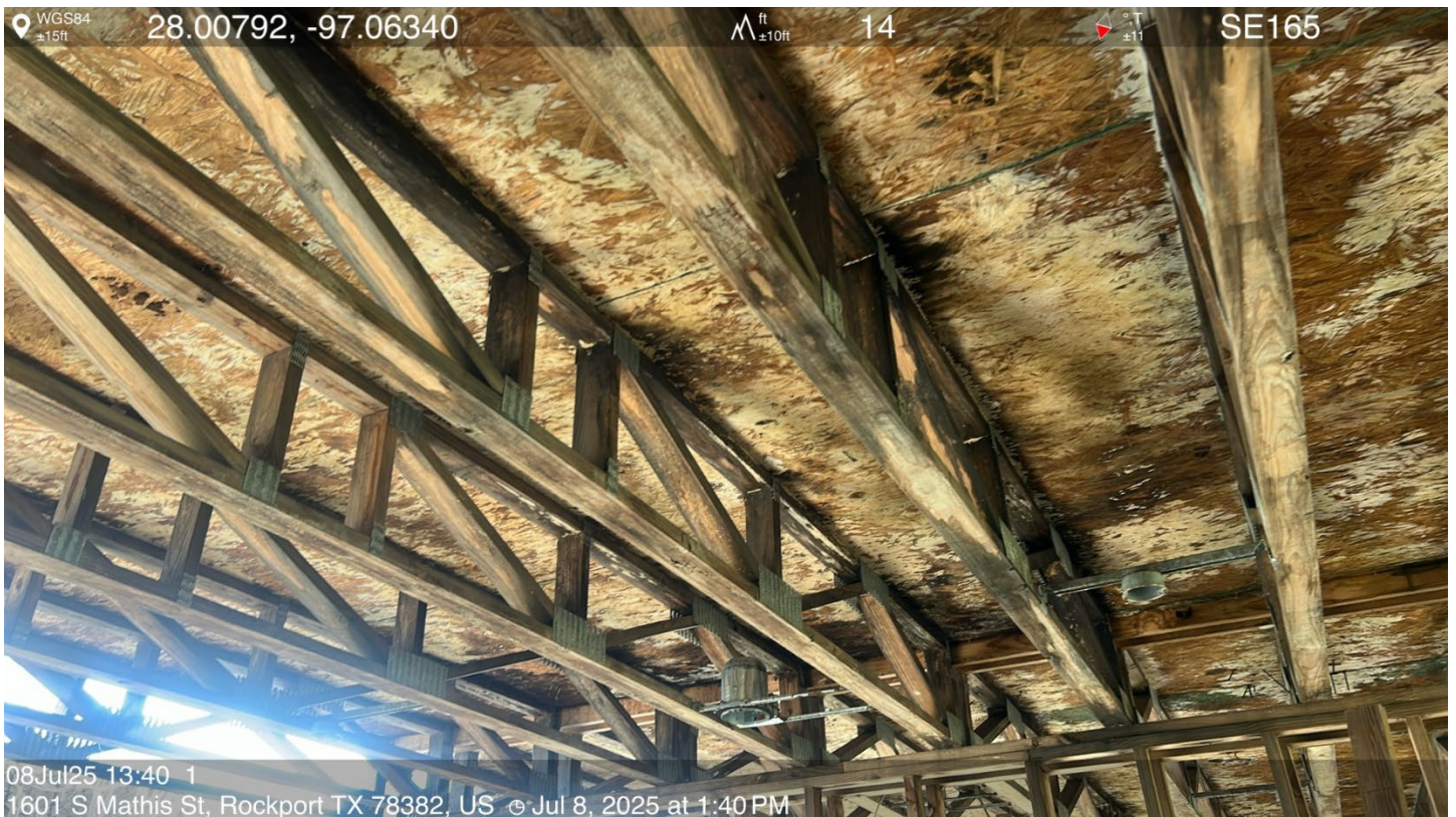
Interior first floor ceiling & rafters
