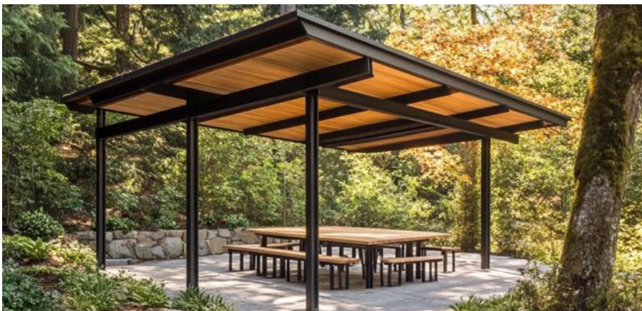
seating pavilion by pond
